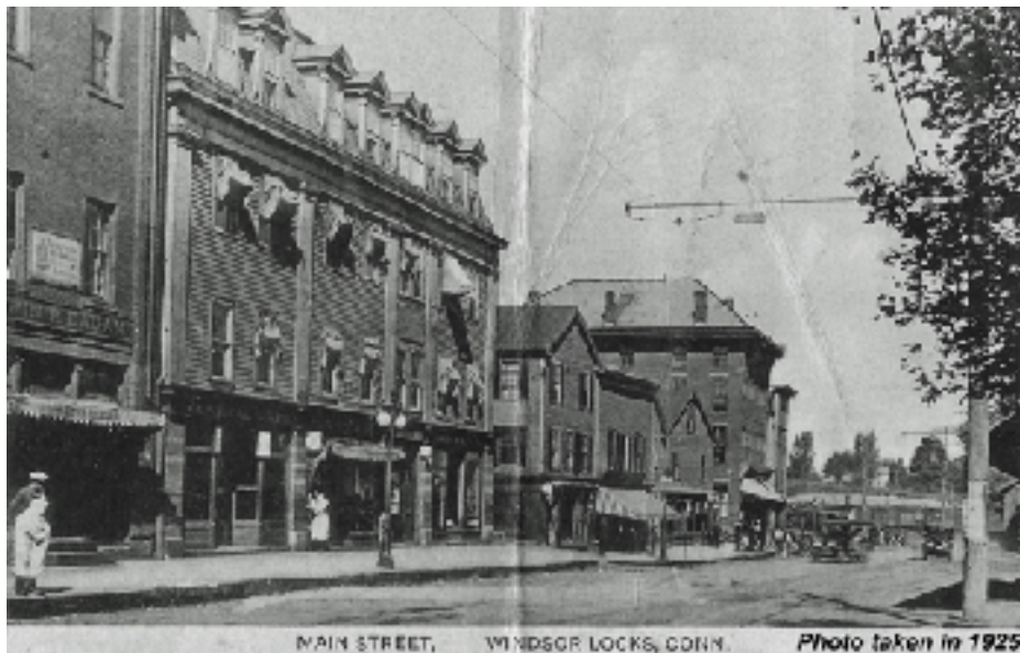
Central Hall block
