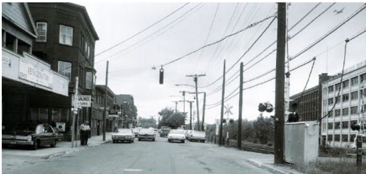
Main Street northbound at Route 140. Canal bridge to the right. 1967
