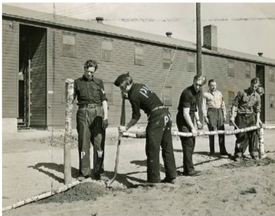
German POWs repairing fence Bradley Field 1944
