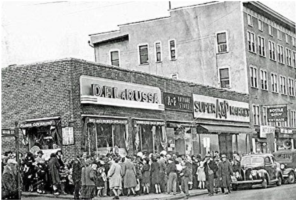
Graziani's Block. The three one-story stores replaced the Burnap Block (also called Central Hall)
