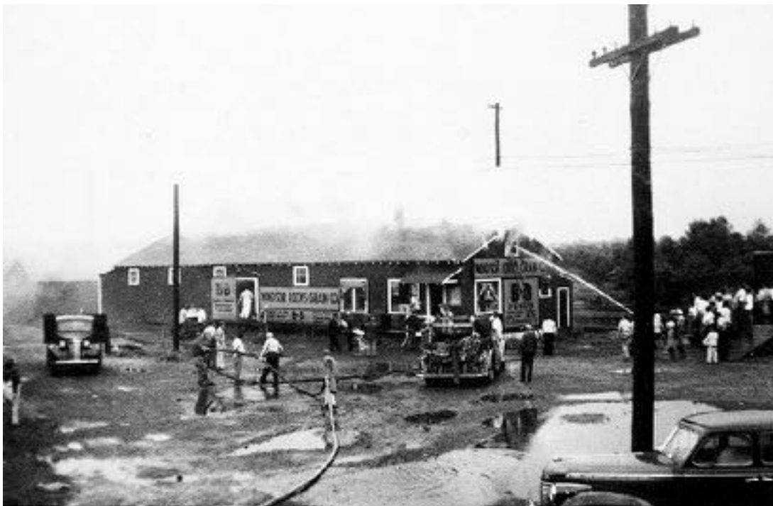
Fire at Windsor Locks Grain Co. June 1947
