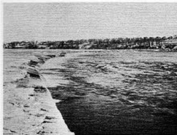
The Dam from the Gate House.
