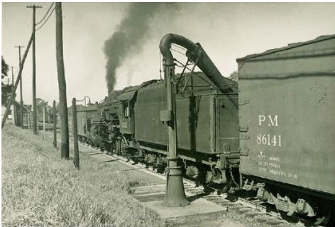
Metal water-tower/spigot near passenger station 1930
