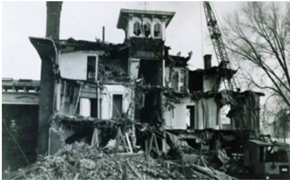
The Ashmere being torn down
