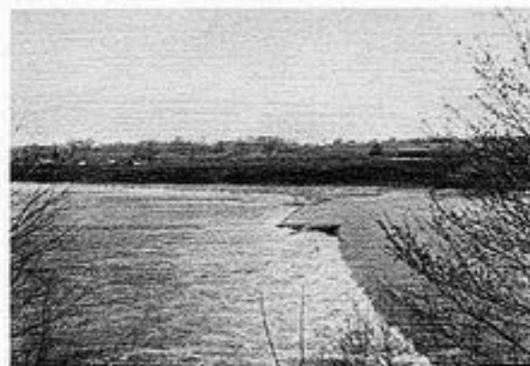
The Dam at Enfield
